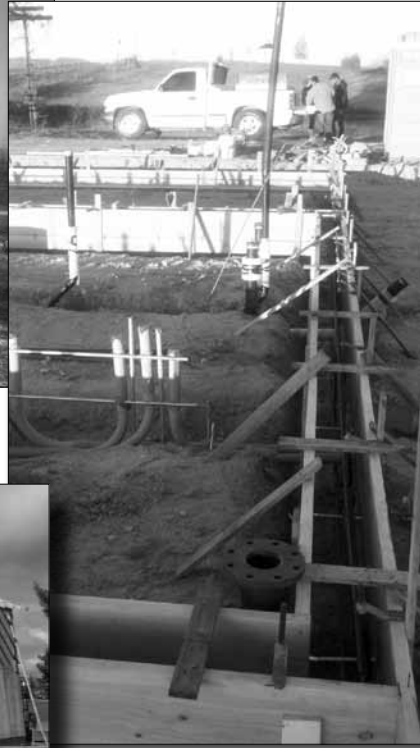
Foundation forms with underground electrical and mechanical (center)
