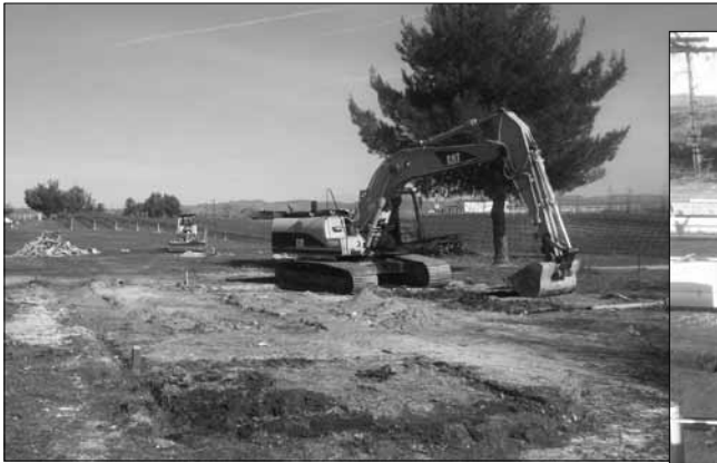
Breaking ground (above)
