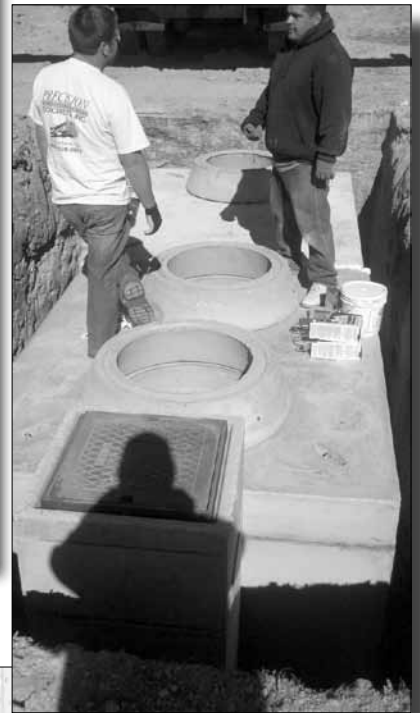
Waste water system clarifier tank (above) for grape juice drains
