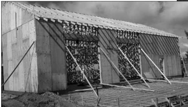
The walls going up! (above and right)
